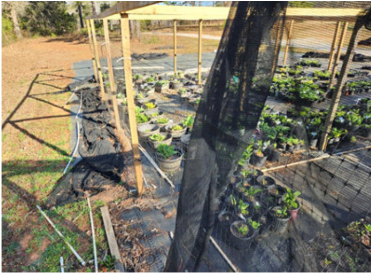
Lumber is anchored in the ground in cement and attached overhead to form a frame for the lightweight shade cloth. Ed uses 50% shade cloth.
